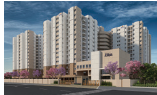
ASHRAYA Bengaluru-Mysuru Expressway Bidadi
